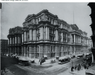
Chicago City Hall and County Building, built 1885. It suffered from structural defects with its foundation that caused the building to sink, and was later replaced with the current City Hall in 1911.
