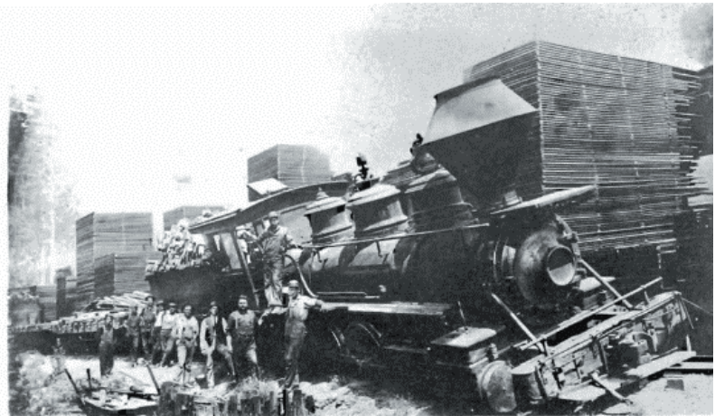
Northwestern Pacific Railroad engine Number 226, 0-6-0, derailed while switching the lumber yard at Navarro.
