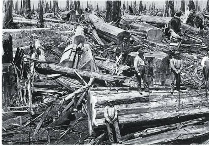
Woodsmen using wedges and jacks to spilt open a log.
