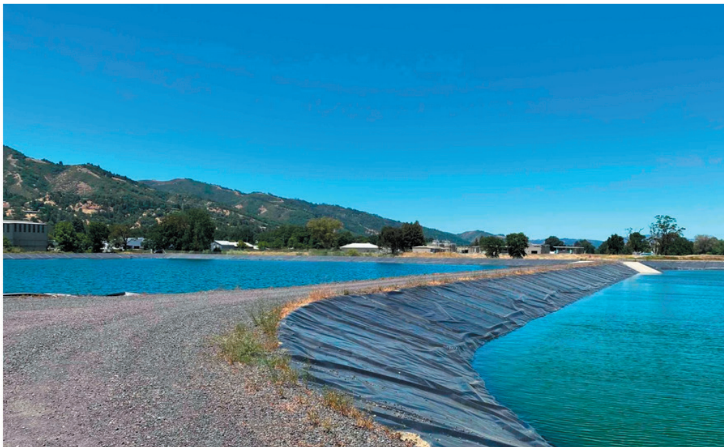
Recycled water storage ponds (Lana Cohen / The Mendocino Voice)
