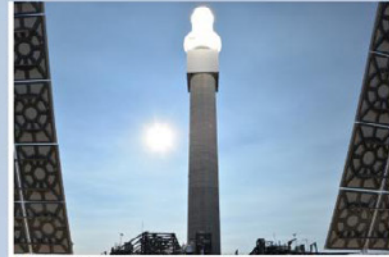
Molten salt receiver is state-of-the-art CSP technology, enabling capturing and storing of the sun's energy, providing reliable electricity on demand.
